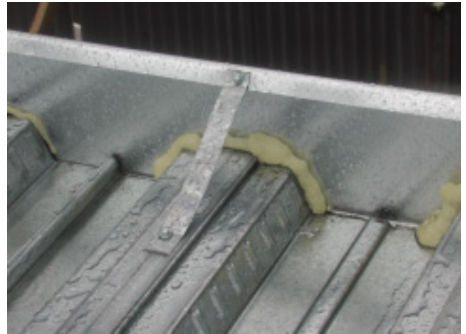
Figure 5: Steel Decking sheets with ends sealed by foam
