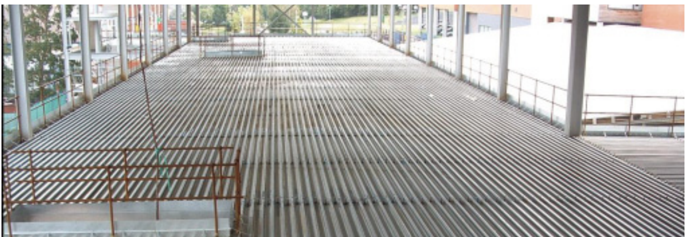
Figure 4: Steel Decking sheets lined through
